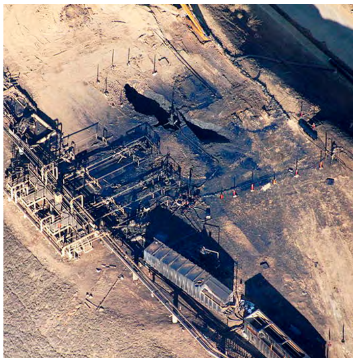
Aerial view of the Aliso Canyon gas leak. Photo © Earthworks, courtesy Wikimedia Commons.
